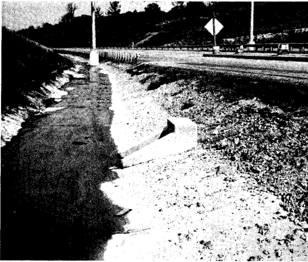
Figure 19. Projecting headwall located within the recovery area.
