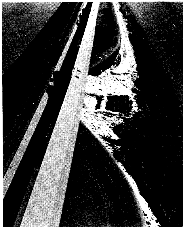
Figure 31. Curb has been curved to direct water to the drop inlet, creating a potential hazard to traffic.
