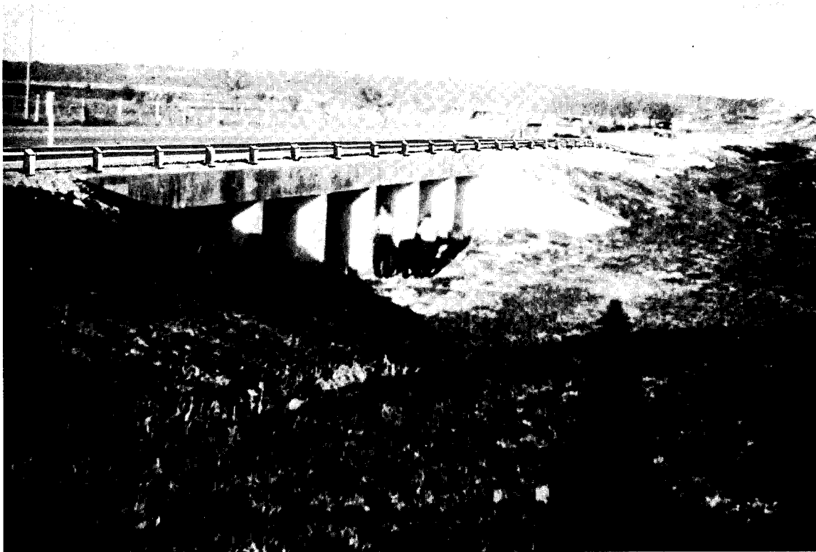
Figure 29. A dangerous situation without recovery area or protection (top). Guardrail installation is the least expensive method of affording some protection to traffic (bottom).
