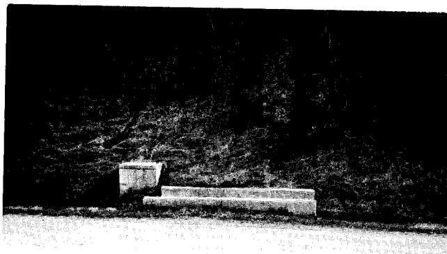
Figure 42. Energy-dissipation devices used to control piped flow from the top of a roadway cut. Both are located near the roadway and are hazards to traffic.
