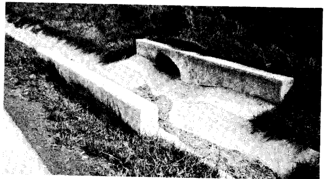
Figure 42. Energy-dissipation devices used to control piped flow from the top of a roadway cut. Both are located near the roadway and are hazards to traffic.
