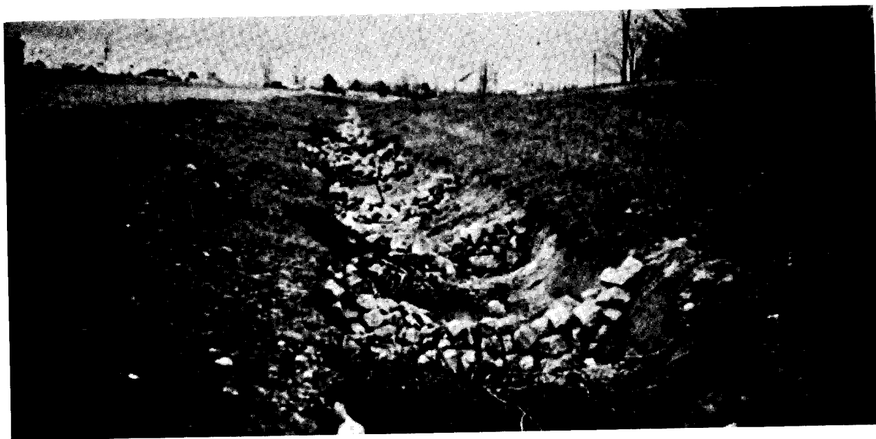
Figure 40. A double hazard: (1) the ditch and (2) the checks that have been placed to stop further erosion.
