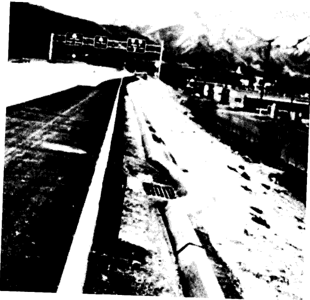
Figure 32. Curb and inlet placed behind guardrail.
