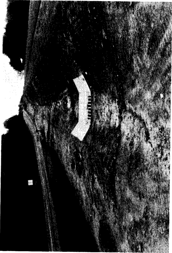
Figure 10. One type of concrete apron to discourage vegetation overgrowth, prevent erosion, and facilitate maintenance.
