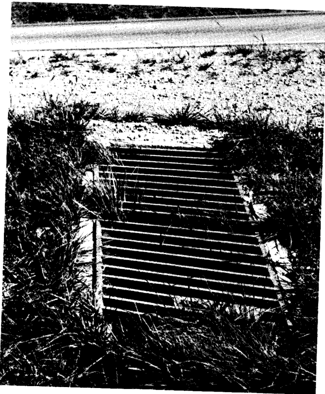
Figure 8. Median drop inlet with grate bars oriented in the same direction as flow.
