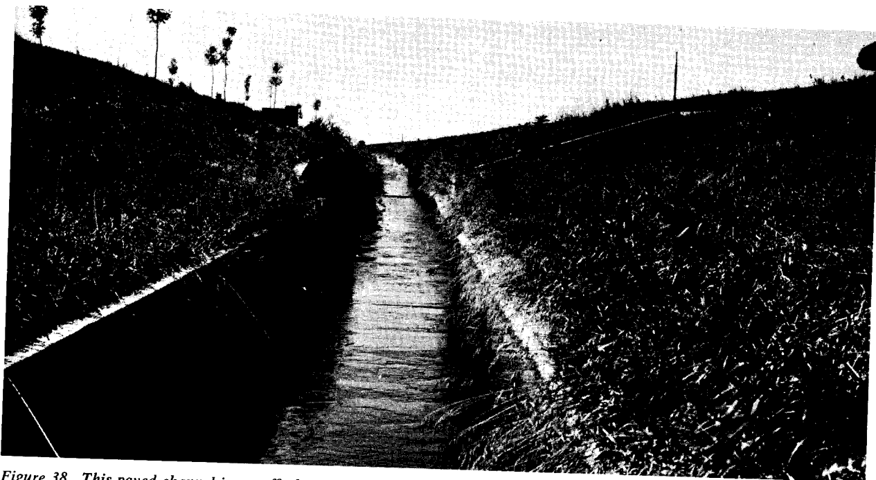
Figure 38. This paved channel is a traffic hazard when located near the roadway.
